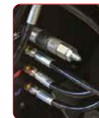
Nitrogen pressure test
